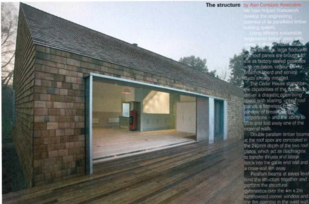
Huge openings puncture the building's reptilian skin. Windows have pronounced galvanised frames which "throw" water clear of the glazing.
