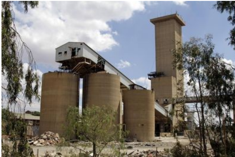
Disused mine buildings and mine access structures at Blyvooruitzicht gold mine
