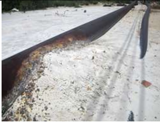
c. Water pollution is ongoing. Please see subjoined.
