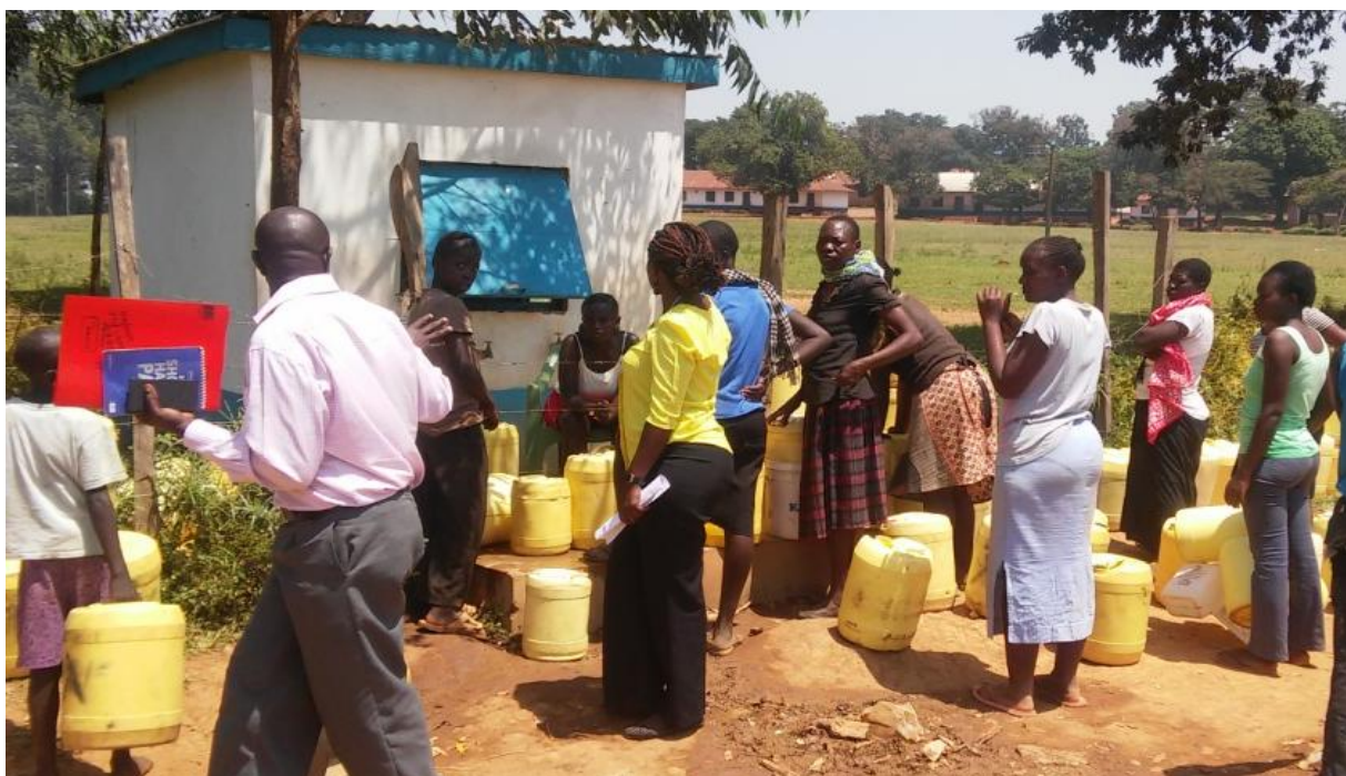
Figure 19: Sidindi Water Kiosk, Sidindi Ward
