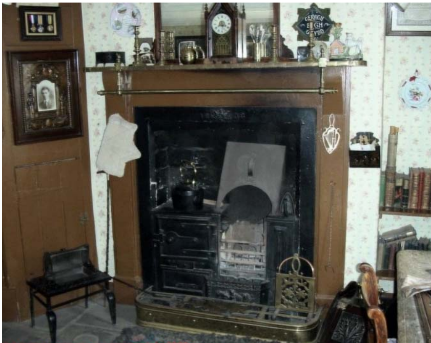
A range identical to the one in my grandmother's house in an almost identical fireplace. It was still there when she was rehoused in the 1970s. When the fire was first lit the metal cover with a handle was held in front of it so air was drawn up the chimney and the coal caught light more quickly. That handle could get very hot!
