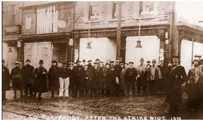
Tonypany residents outside the damaged shops
