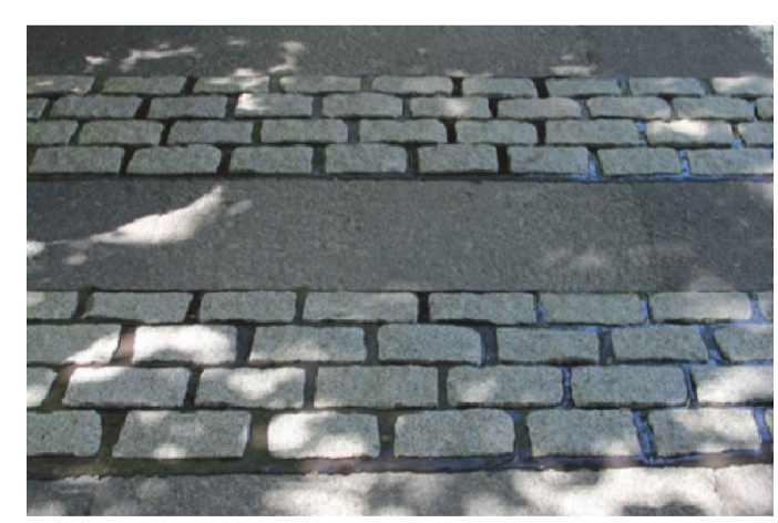
Quickset Rumble Strip Detail
