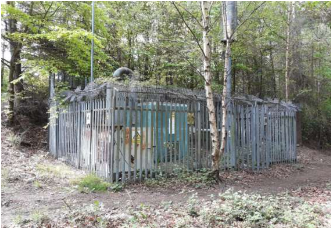
Image 2 - Existing Landfill Gas Plant Compound
