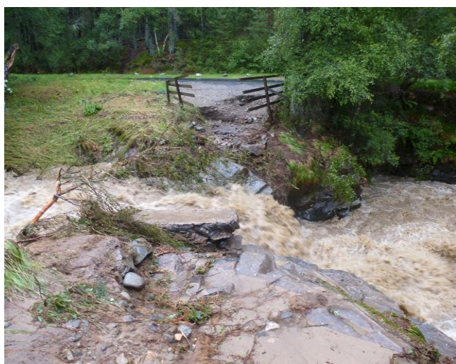
The site of the bridge on the morning of 11 th August 2014
