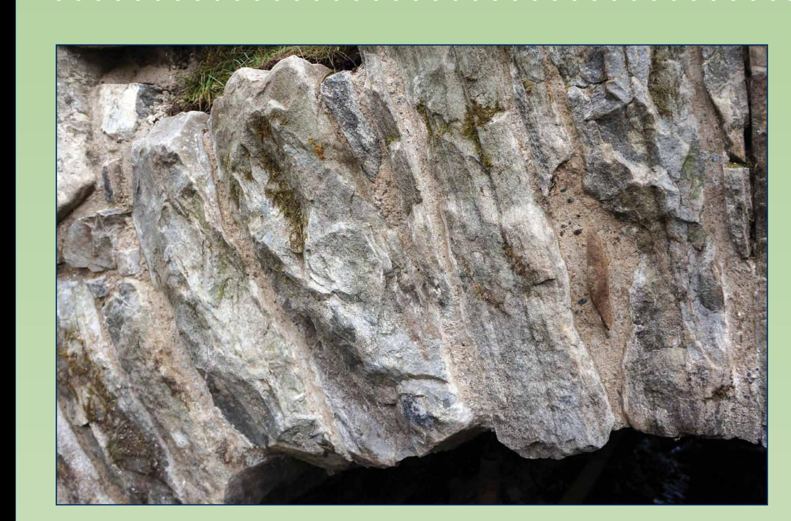
The three single-span humped-back bridges at Achlain were consolidated and expertly repointed with lime mortar by Graeme Brown Stone Masons Ltd under the direction of Krystyna Pytasz from Addison Conservation + Design. This is a detail of repointed voussiers from the south face of the central bridge.
