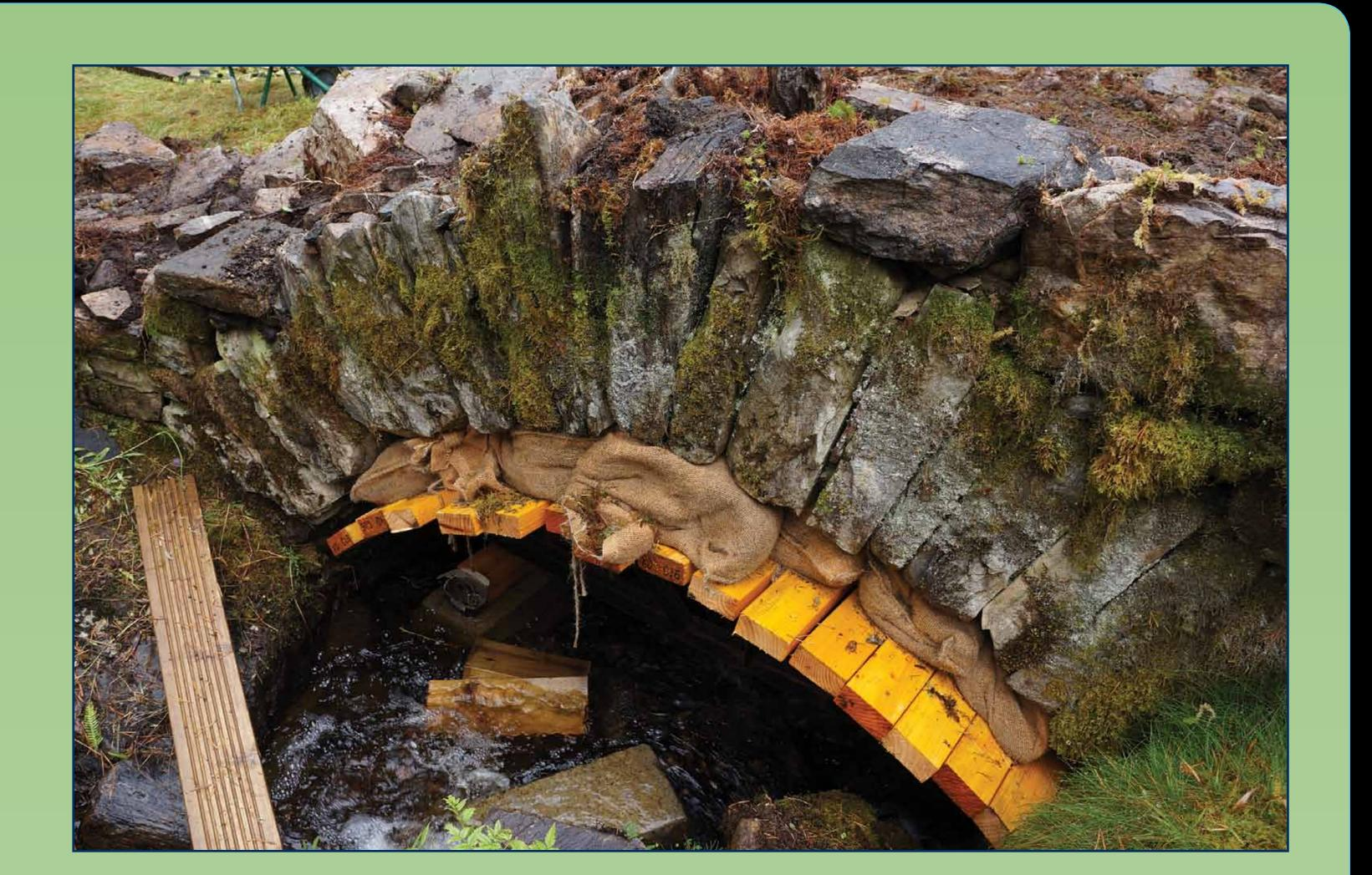
The core of the arch comprised upright voussiers pinned and locked together with small slabs and packed with sand and gravel at the surface. The voussiers and smaller pinning slabs were also clearly visible in the underside of the structure, with gaps evident where slabs had fallen out. The stone masons supported the arch with a steel frame, timber and sandbags, realigning slipped voussiers and repining them from above.
