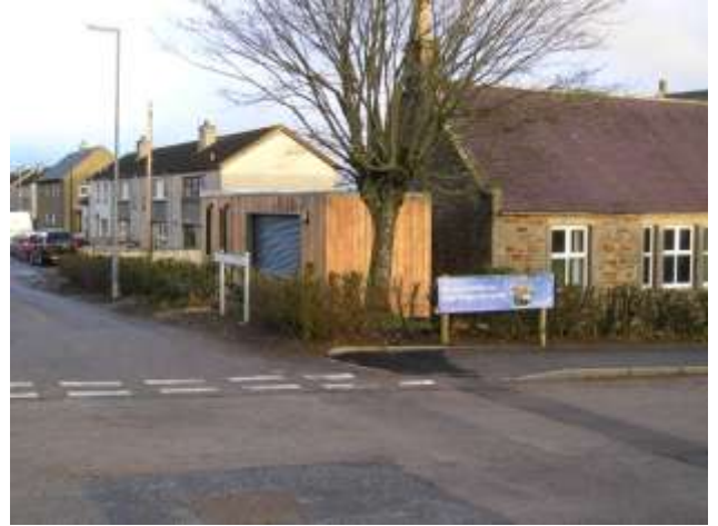
The New Cabin on Site
