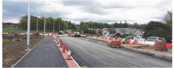
Three lanes to increase the volume of traffic going through the crossing. The same layout is on the other side of the junction, giving a total of five lanes.
