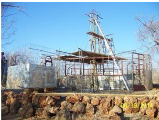
immediately put to work helping install support for the brick water tank floor. The plan is to harvest large amounts of rainwater and thus demonstrate the value of water harvesting but also to save US\$12,000, which would be the cost for a borehole, not to mention the continual maintenance cost.
