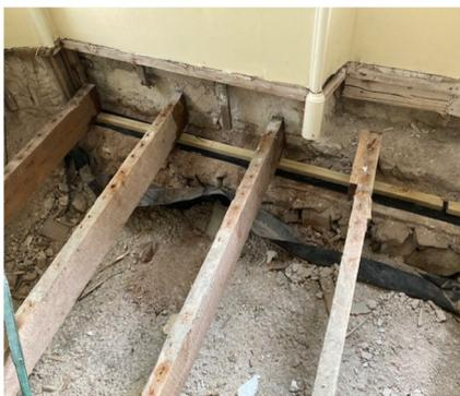
When digging around in an old house you have to expect to find some previously unseen issues. This pic shows that the wooden plates on which the joists rest were rotten in places so I replaced these where necessary. These pics show the rotten wood removed and then the joists resting on new plates underneath over damp proof strips. You can also see the lath and plaster wall construction and the lath battens onto which the skirting board was fixed - all in good shape.
