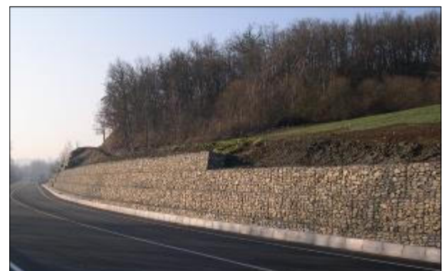
Example of gabion wall
