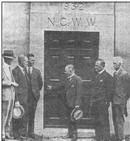
Alderman A. R. Atkey, chairman of the Water Committee, unlocks the door of the pumping station.
