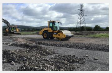
Once we've completed the road accesses, we start to build the construction haul road
