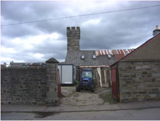
Castellated chimney, corner of Chapel Street and Market Street
