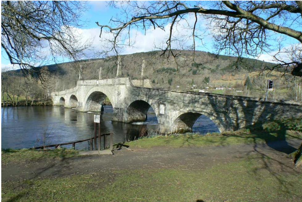
General Wade's Bridge over River Tay
