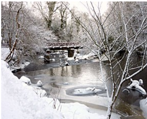
Redhall Bridge just downstream from the weir
