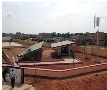
A self-sustaining water filtration system at the University of Kenitra in Morocco. Solar panels and a wind generator power the system that is visible under the right-most solar panels. From there, fresh drinking water is delivered to the taps in the foreground. (Credit: Firmus)
