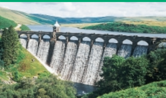
Elan Valley Hydro Scheme Hyder, in response to NFFO, has successfully developed 5 separate yet interconnected hydropower schemes in the Elan Valley, Mid Wales.
