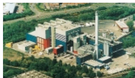
Tyseley The 25MW energy-from-waste plant at Tyseley, awarded a contract under the NFFO-3 round, uses well-established technology to turn 350,000 tonnes of Birmingham's waste per year into electricity.
