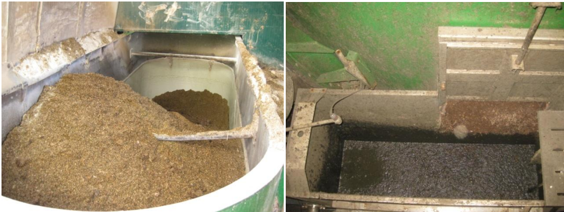
Picture 6: Solid substrate feeding (left) and mixing unit (liquid + solid)
