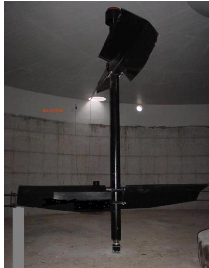
Picture 9: Slow going agitator in F1 (left) and vertical decentralized placed slow going agitator (F2)
