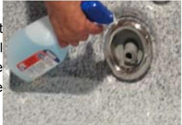
2) Soak jet inserts in a mixture of 1 part vinegar to two parts warm water for 2-3 hours. Periodically rotate the spinner nozzle to break up residue in the jets.
