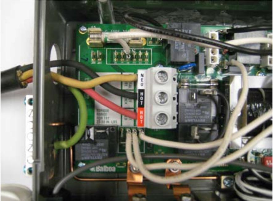
Connect each color to its respective terminal block location. The Ground (green) wire must be connected to the grounding terminal which is outside of the System box. The Grounding wire must first enter the system box and then access the grounding terminal via a hole on the side of the box adjacent to the grounding terminal as shown in the picture above.
