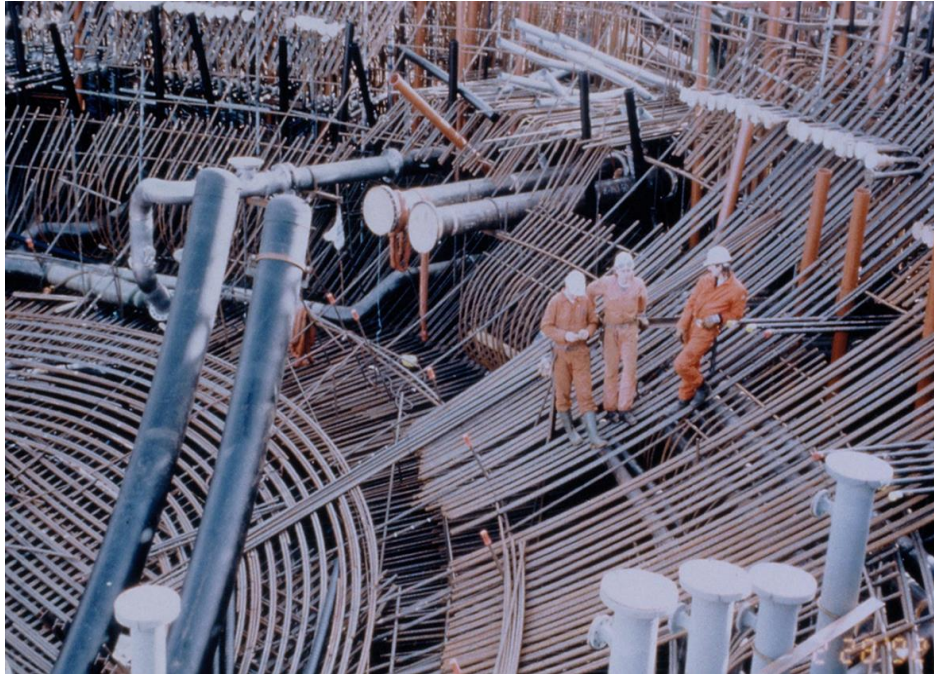
Rebars and piping systems prior to concreting
