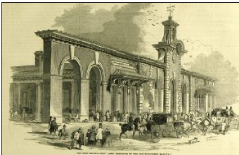
UNDER CONSTRUCTION: The Bricklayers' Arms terminus, pictured in May 1844
