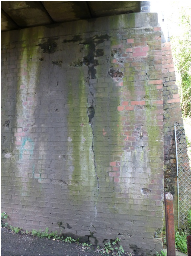
Figure 50 – Spalling and hairline full height fracture (<5mm) to high mileage abutment. Vegetation requires removal from structure and treating to prevent regrowth.
