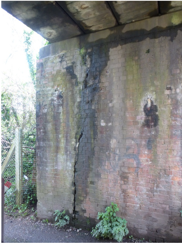
Figure 51 – Spalling and full height vertical fracture in low mileage abutment (<25mm). Stepped hairline fracture visible at top of the abutment.
