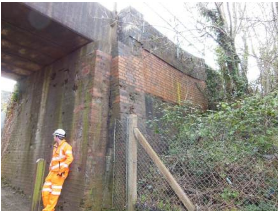
Figure 49 – Spalling to masonry on buttress and abutments
