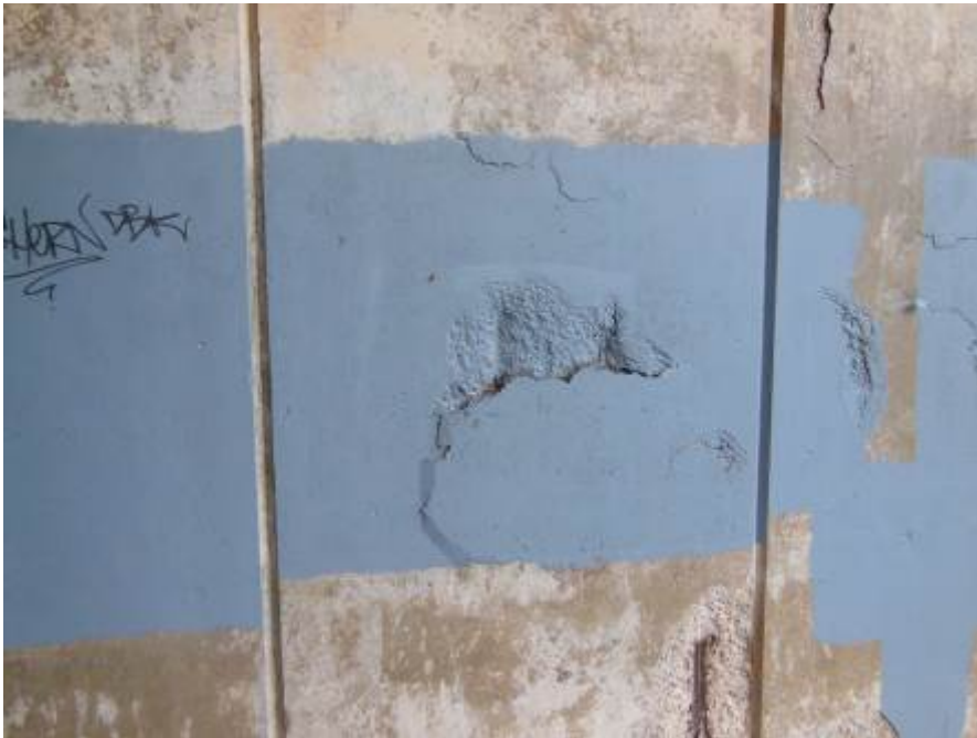
Figure 44 - Spalling to the abutments
