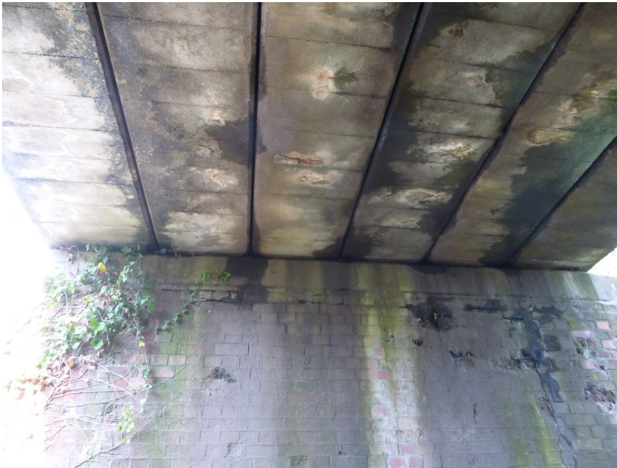
Figure 48 – Bridge soffit: isolated spalling and visible corrosion
