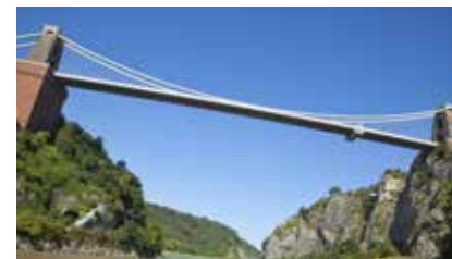
4 Clifton Suspension Bridge
