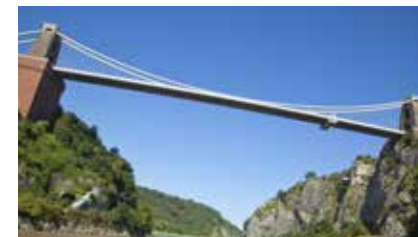
4 Clifton Suspension Bridge
