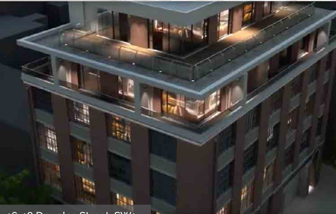
16-18 Douglas Street, SW1
