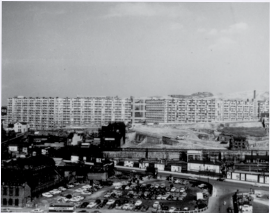
Park Hill under construction, circa 1960 – a dramatic new presence on the Sheffield skyline.
