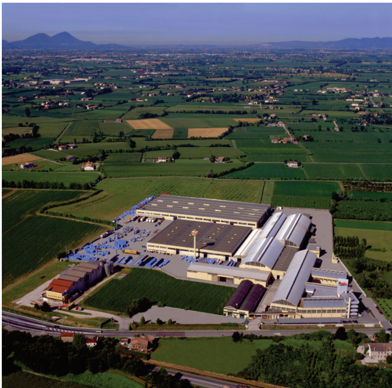
Headquarters and main plant - Limena (PD)
