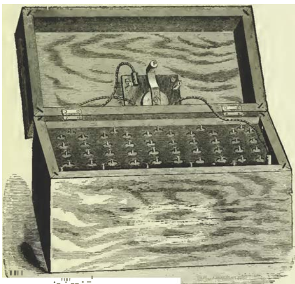
FIG. 20.-SILVER-CHLORIDE BATTERY OF FIFTY CELLS.
