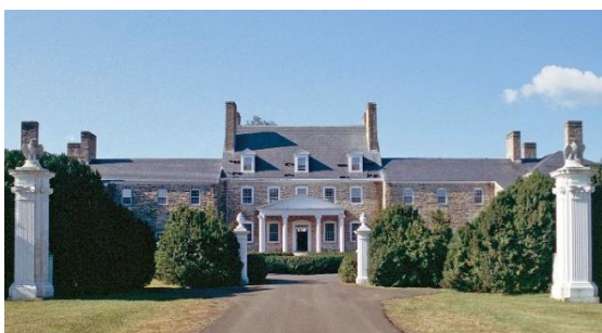
30. North Wales in Fauquier County, Virginia, built for William Allason between 1776–96 Image courtesy Virginia Dept. of Historic Resources © Cheryl Shepherd, 1998
